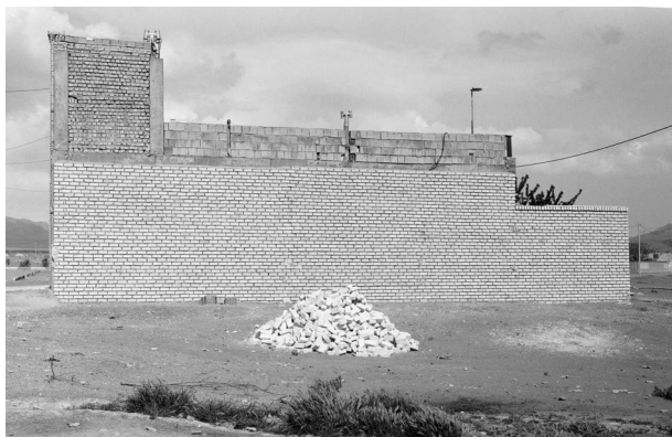
Found Installation No. 63
