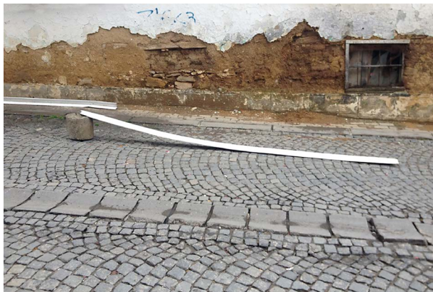
Found Installation No. 41
