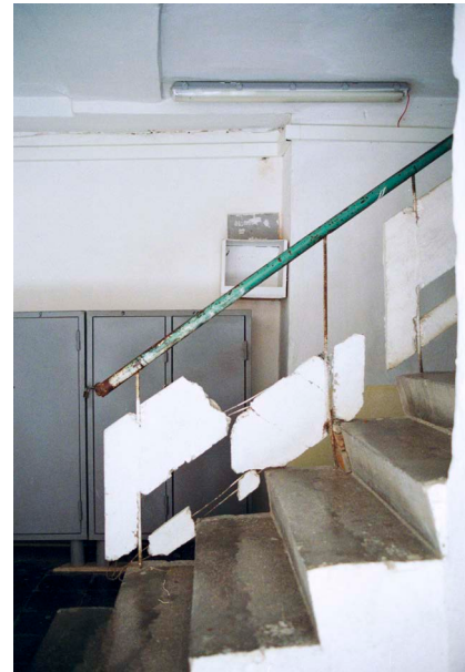
Found Installation No. 34
